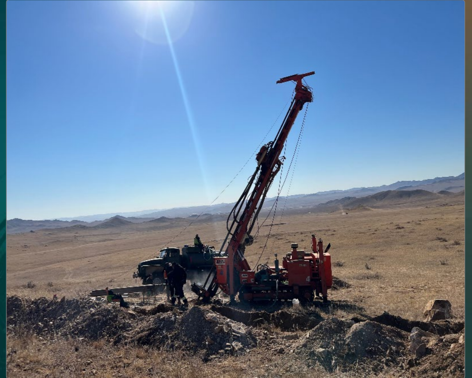
Nukht exploration site NUKTH-01 borehole, NUTTR-02 excavation channel
